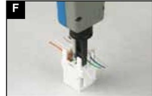
**F** Terminate wires using Linkbasic tool (P/N: TLA11) or equivalent.
