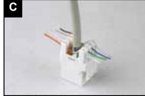
**C** Insert each wire into the appropriate channel according to the color code on the module, keep the cable perpendicular to the block.
