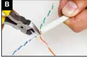
**B** Fan out cables based on desired wiring scheme, cut the pair separator and rip cord(if present) as close as possible to the jacket. Note: Be careful not to nick conductors.
